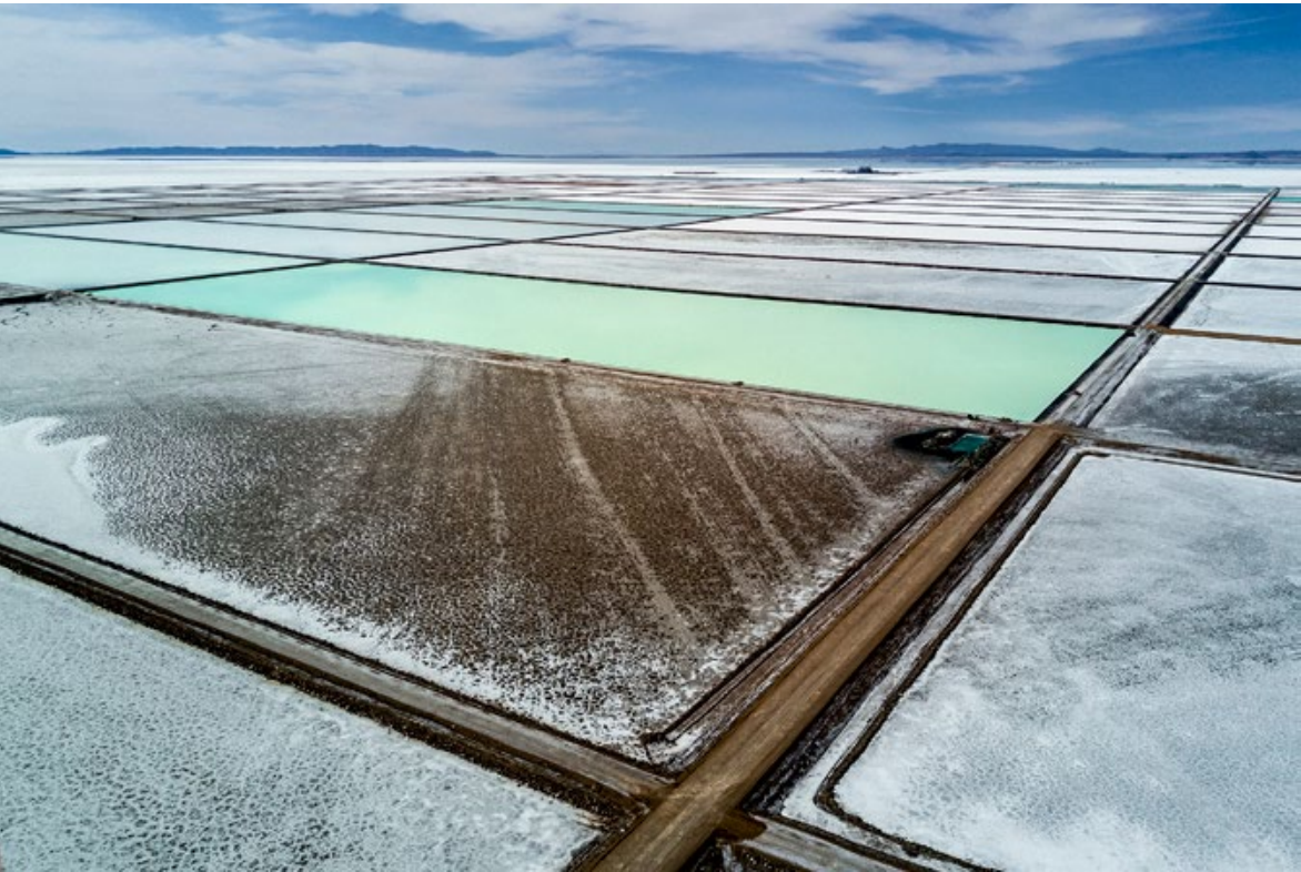
Enormous lithium pools near Llapi production plant. Brine is pumped into these large evaporation pools on the southern edge of Salar de Uyuni, where it is left to evaporate for many months. It is then processed at Comibol's Planta Llapi nearby.
